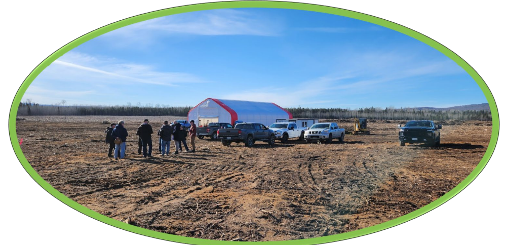
Lake Nipigon RNG and Biocoal Facility Site March 2024
